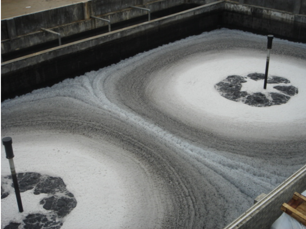
Photo 2: Self-entrained Jetox venturi aeration provides for efficient mixing and prevents sludge settlement
