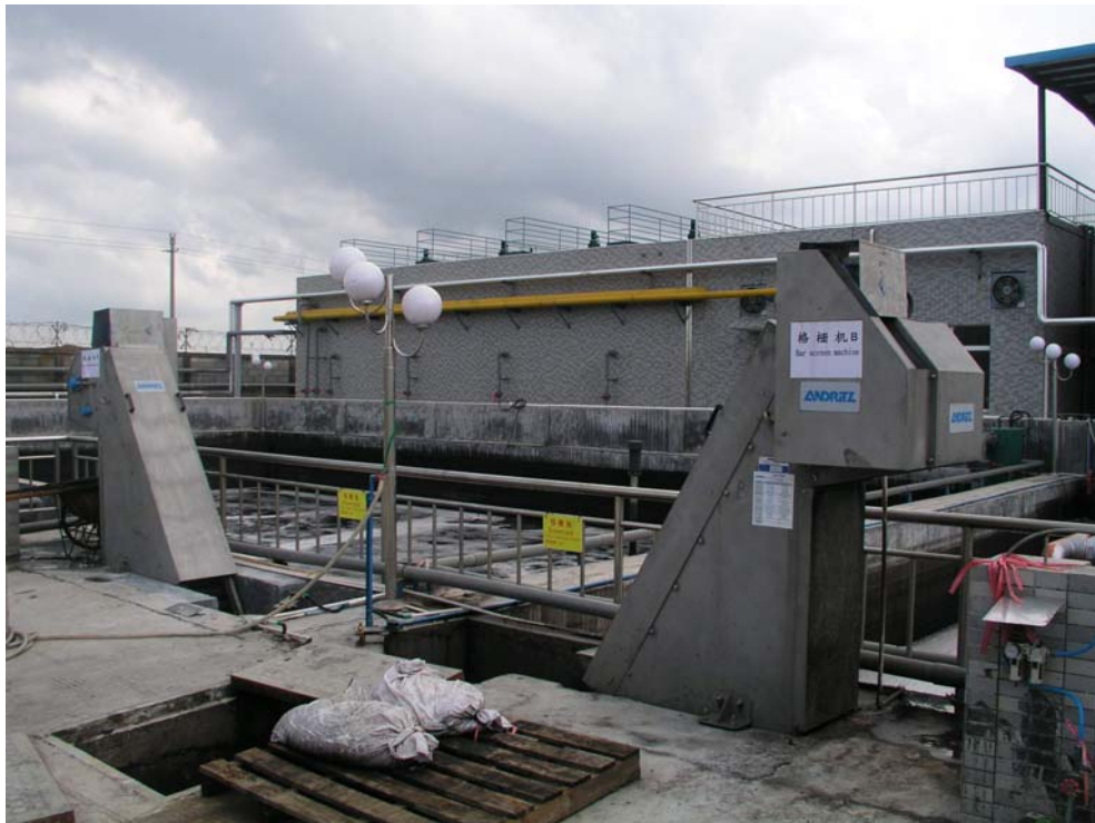
Photo 1: A fully automatic self-cleaning screen with 1mm slot size provides for adequate pre-treatment
